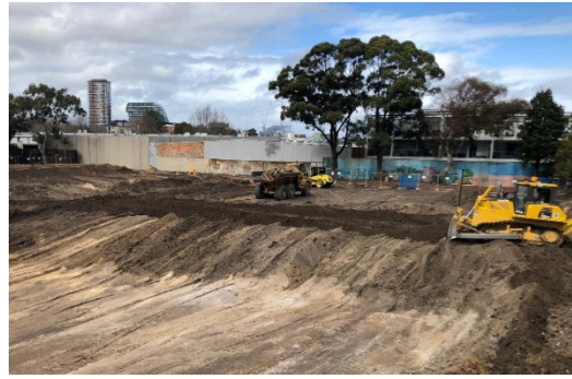
Caption: Earthworks on site
