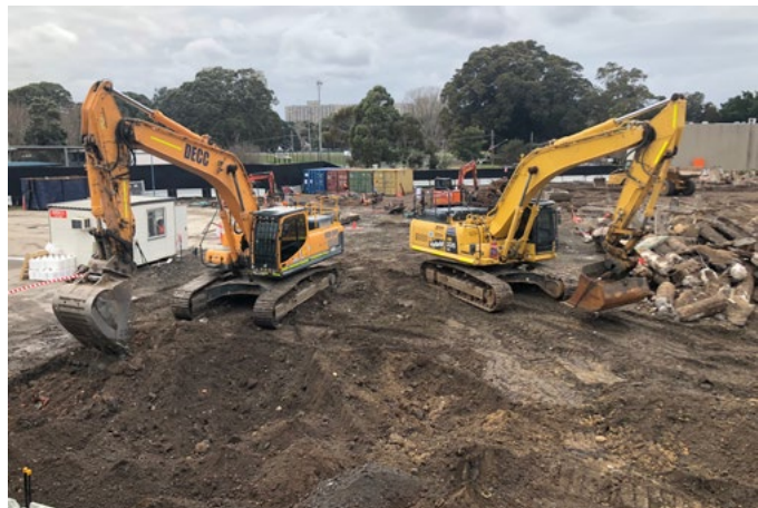
Earthworks on site
